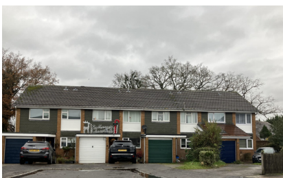
Terraced row with slate, pitched roof
