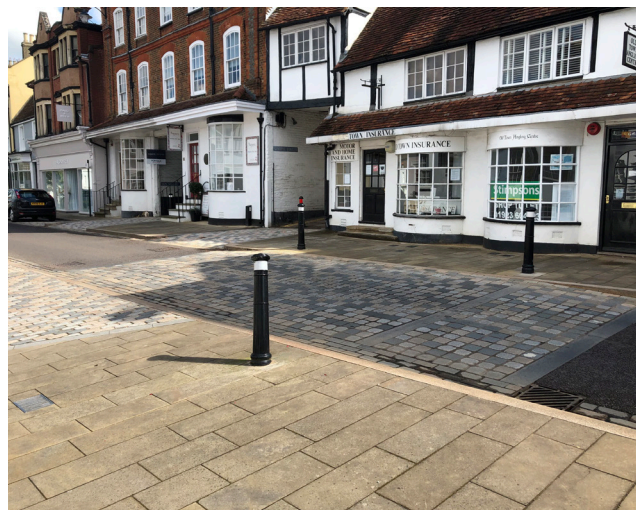
Figure 36: An example of raised pedestrian crossing with a plateau in Hemel Hempstead.
