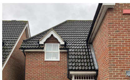
Jerkinhead roof with small gable dormer featuring black pantiles
