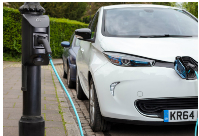
Figure 33: Example of on-street electric vehicle charging points. Source: www.theguardian.com .
