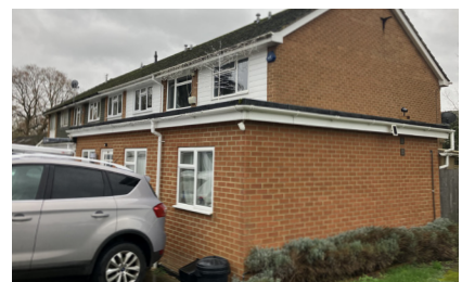
Flat roof garage extension
