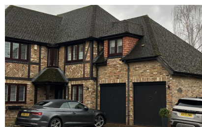
Intersecting hipped roof
