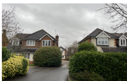
Pitched roofs with intersecting hipped fronts and gable dormers
