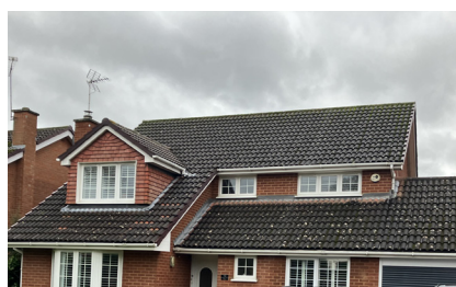
Slate pantile, pitched roof with gable dormer
