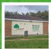
Solar Panels for the Pavilion and more!
